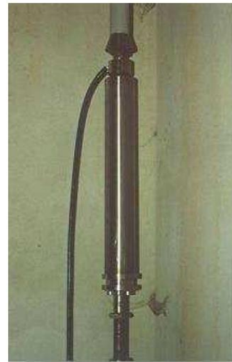
Seismic retrofit of the bell tower of the church of San Giorgio in Trignano (DesRoches and Smith, 2002 )
